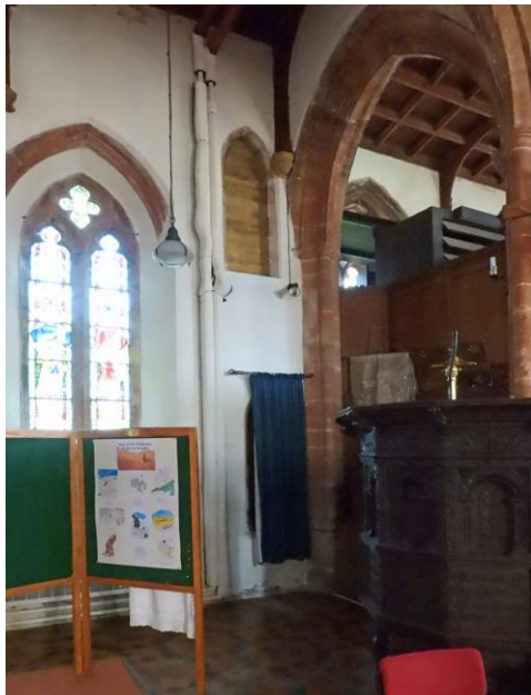
The blocked-up entrance to the Rood-Screen
